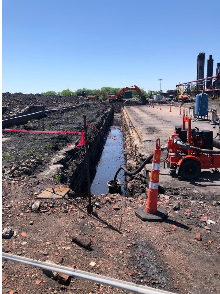
Photograph No. 1 – Exhaust Tunnel Looking West, After Removal of Tunnel Roof
