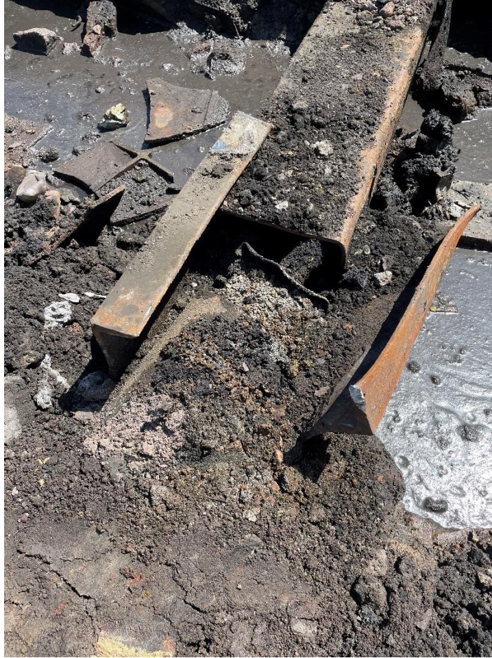
Photograph No. 2 – Rectangular Beam with Vermiculite Fill
